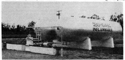
against contact with truck and trailer in handling into filling position. The electric control switch and the vapor return valves are seen mounted at the top of a central concrete pillar, while liquid hoses for simultaneous attachment to truck and trailer are supported, as can be seen, over the top of the concrete wall with attachment valves laying in Y supports at either end.
